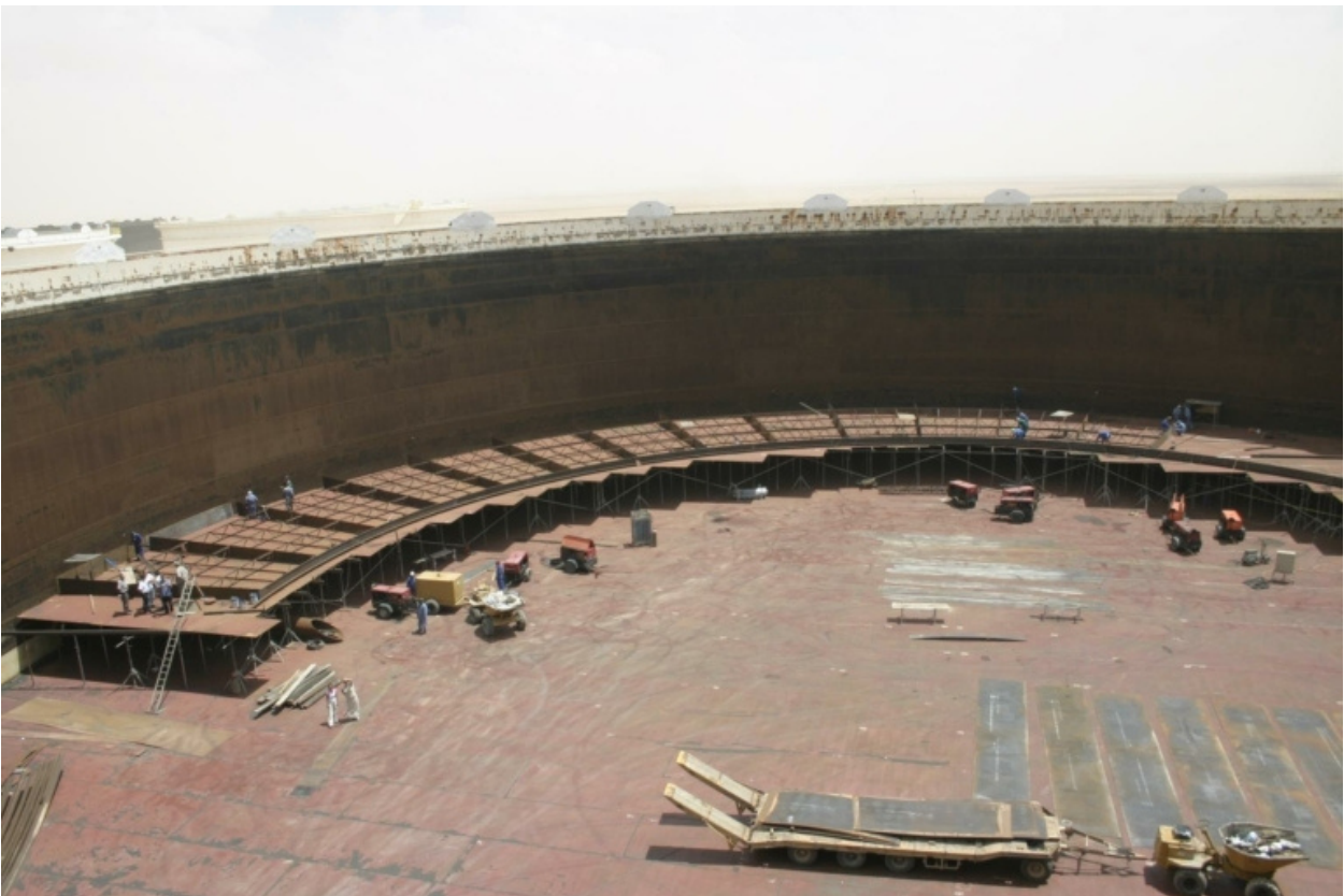
Image 1 Crude Oil Storage Tank External Floating Roof Site Erection
